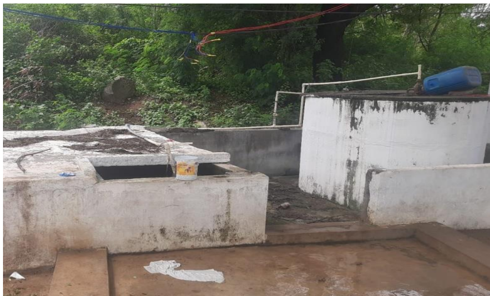
RO waste water storage sump
